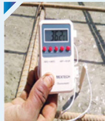
Measuring temperature of concrete during extreme weather conditions
