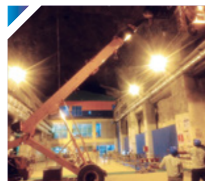
Earlier: T.G HALL with conventional lightnings at Dikchu HEP
