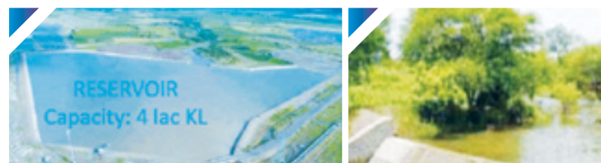
Reservoir and check Dam construction at ghani solar park
